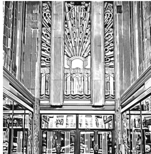
Figure 3: Detail of main entrance at the Eastern Columbia Building, Los Angeles
