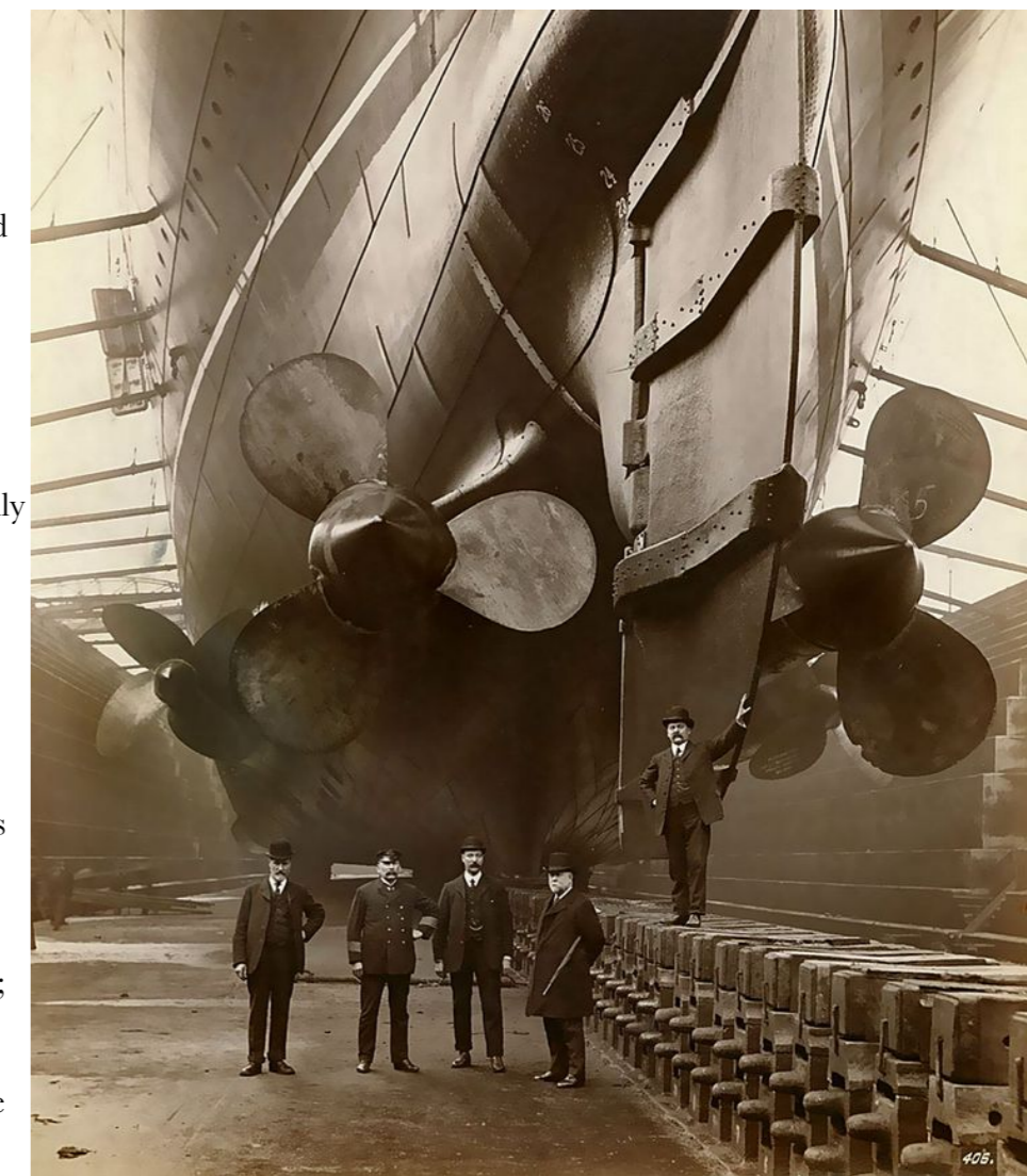
The Lusitania had four screws, with one boiler room and one funnel for each—unlike the Titanic which had only three screws but was given a fake fourth funnel
