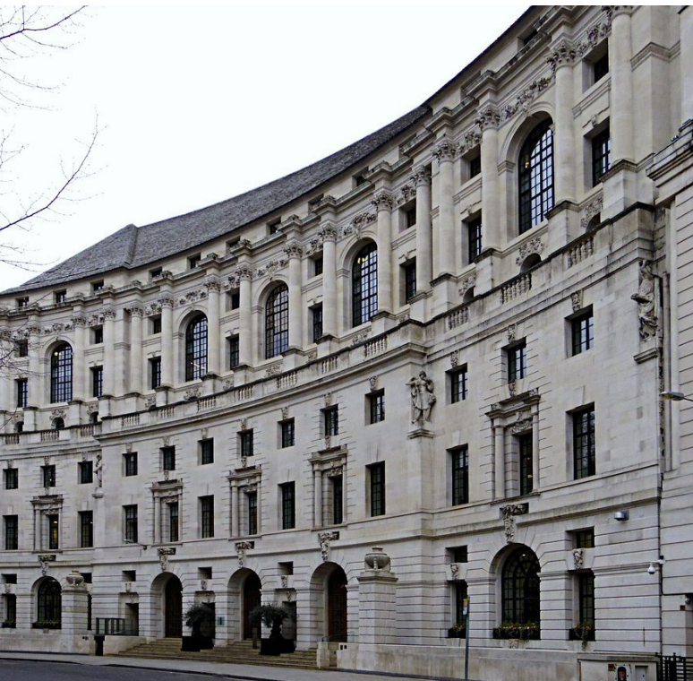
(Above) Lutyens's Britannic House (1920) shows the movement towards a restrained yet monumental classicism, later to be known as "stripped classicism"; (below) A 1960s addition to the iconic Chartered Accountants' Hall mars it with clashing, brutalist hammered concrete fabric; (below right) a 1988 addition to the Royal Exchange (the top storey) is admirably indistinguishable from the existing period
