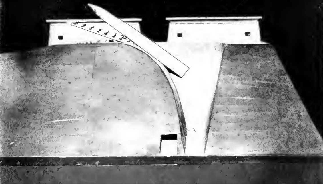
In The Problem of Obelisks (1923), English engineer Reginald Engelbach proposed several obelisk-raising ideas. One theory involved dragging an obelisk up a ramp using rollers and a sled and lowering it down into a funnel-shaped pit where, aided by stabilising ropes, it came to rest on a pedestal
