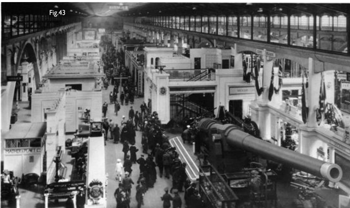
Interior Palace of Engineering BRITISH EMPIRE EXHIBITION, WEMBLEY.
