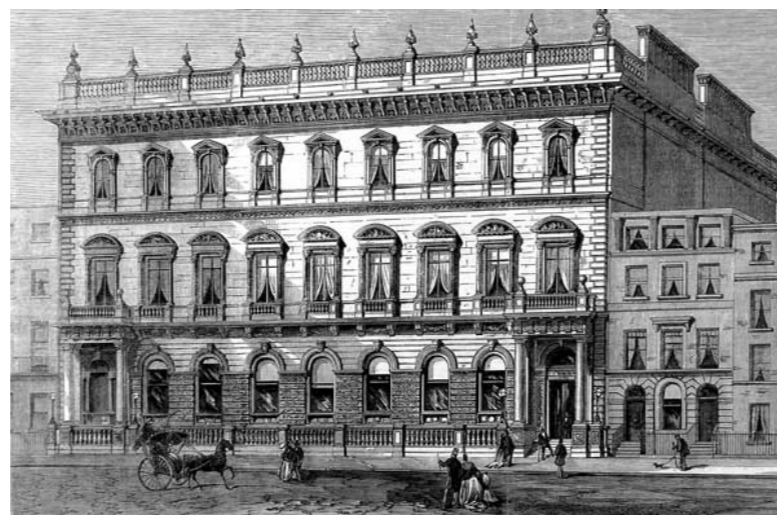
The Junior Carlton Club, 30 Pall Mall, from the Illustrated London News 1868. The Carlton was at No.96; bombed in the war, its site proved difficult to sell so the Junior Carlton moved there. However, a decision to rebuild as a modernist "club of the future" in 1968 drove away most of its remaining members at it wound down in 1977
