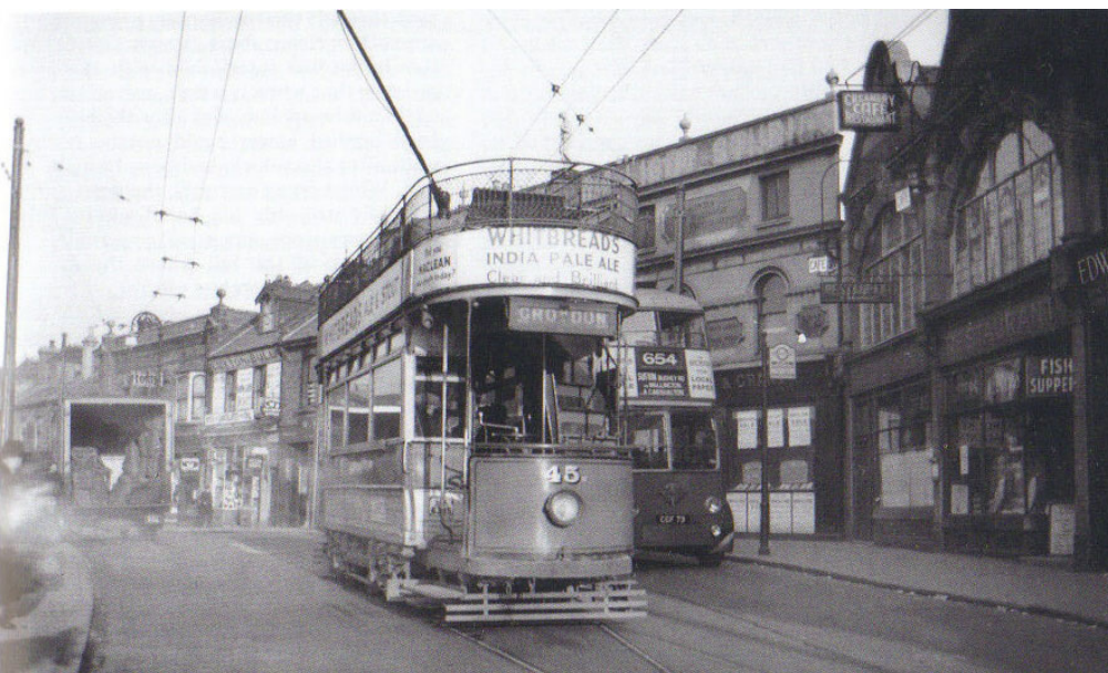
A time of transition. Route 654 is currently working only between West Croydon and Sutton, and at the former point no.73 squeezes past former Southmet tramcar 45s newly arrived from Crystal Palace. The contrast between the brand new trolleybus and the British-built four-wheeled open-topper of 1906 could hardly be greater.
