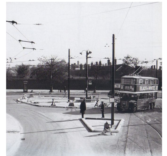
A new roundabout was constructed at Hampton Court in time for the start of the 667 whose wires lead off towards the camera. Air-brake-equipped Diddler 60 is seen circling the new wiring at the start of a Wimbledon journey on the 604
